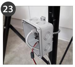
Mount the control box and cables, but don't connect power until setup.
